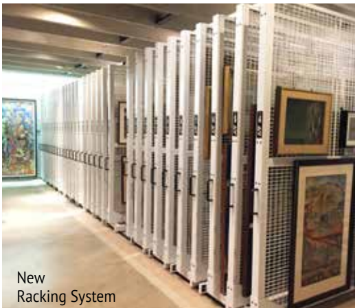
Installation In Process
